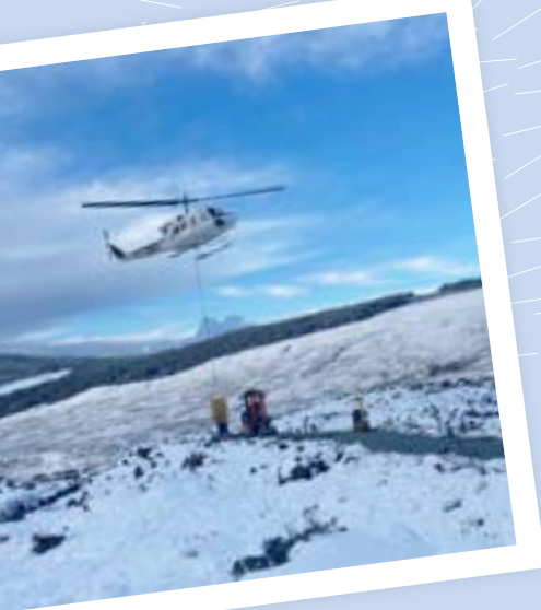
A HELICOPTER DELIVERS MATERIALS FOR THE FAIRY POOLS PATH TO CONTRACTORS
