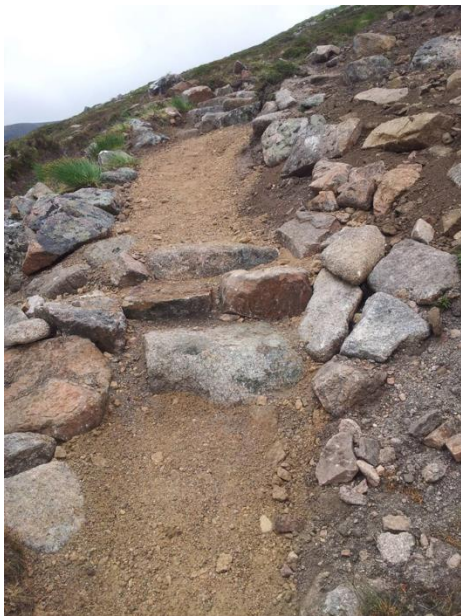
Hand Built Aggregate Path
