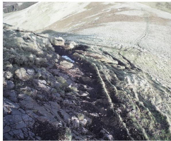
Steeper eroded slopes requiring hand build only due to steepness of the terrain
