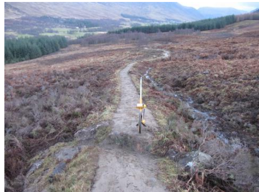
Raised machine path with turve side drain at Angus Glens (Cairngorms National Park)
