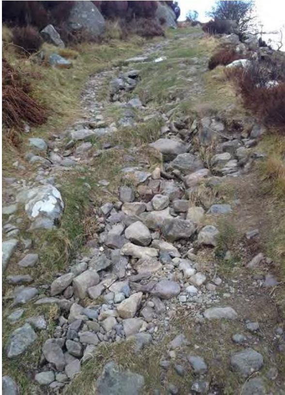
Figure 1 and 2 – Built surface breaking down on zig zags due to collapse of drainage systems
