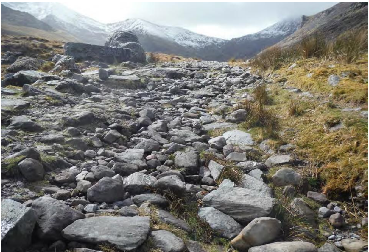
Figure 2 - Surface Loss and Drainage Problems
