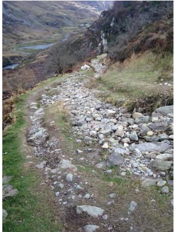
Figure 1 and 2 – Built surface breaking down on zig zags due to collapse of drainage systems
