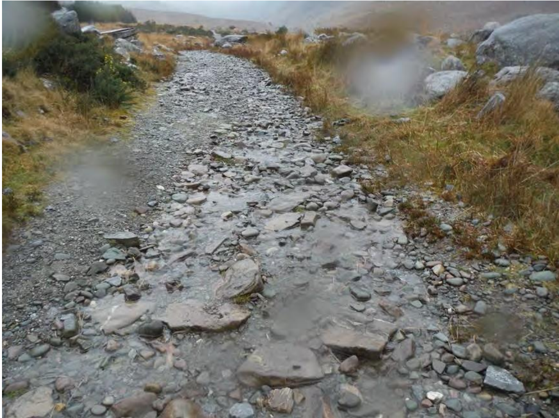
Fig 1 – Lateral Drainage required on section 1
