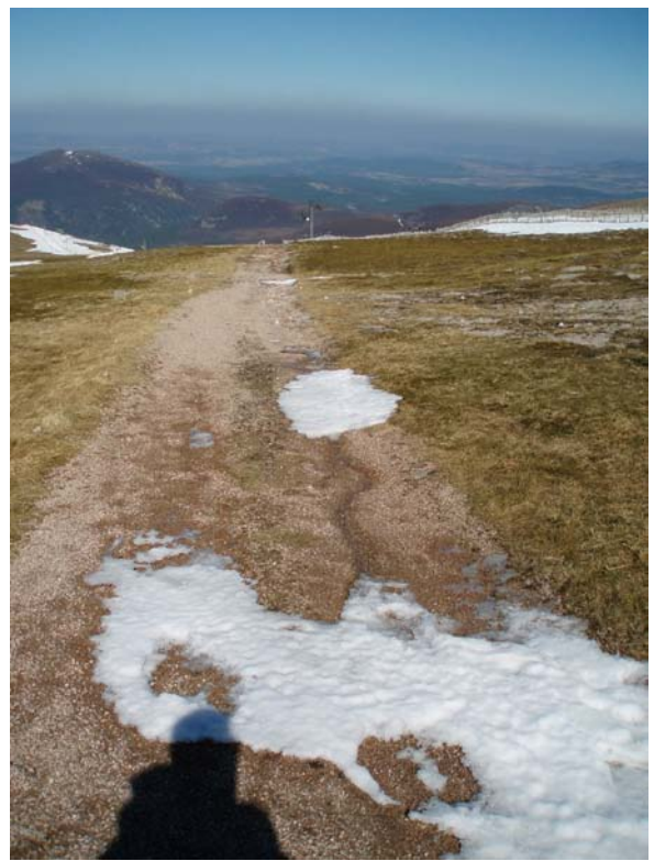
Some rilling of loosely bound materials.
