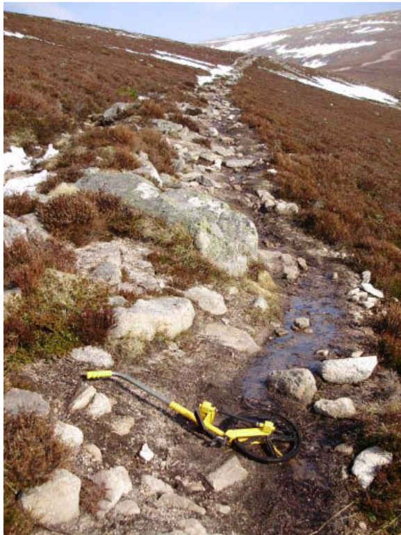
Section 3 – path line gradually migrating down hill.
