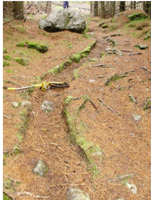
Some gullying on steeper sections.
