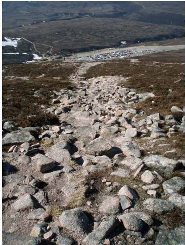
Some rilling of loosely bound materials.
