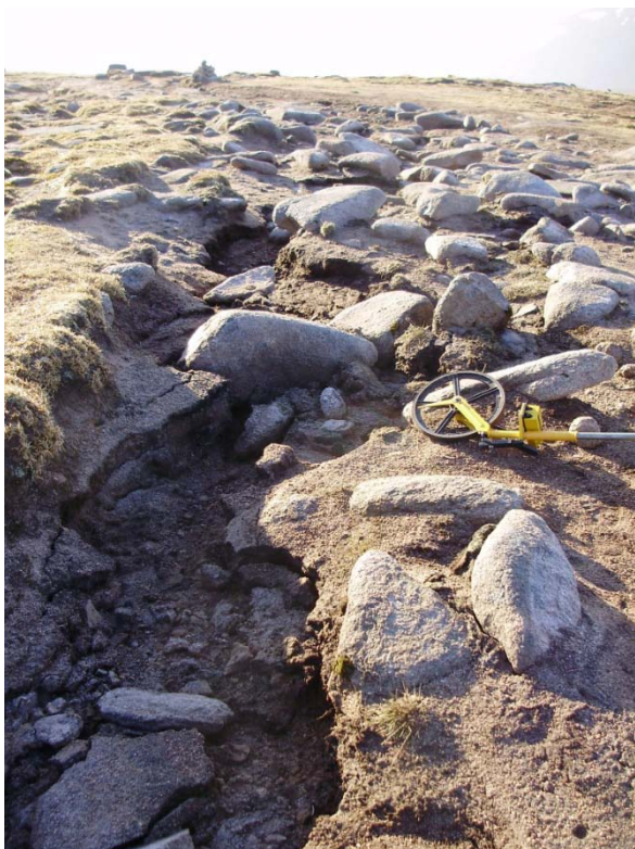
Some gullying of fines where unprotected.
