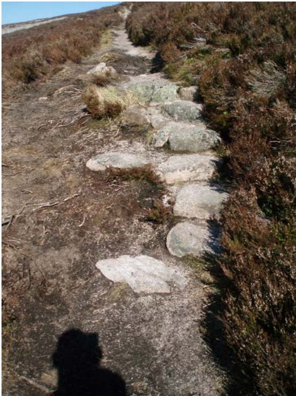
Path spread on easier gradient.
