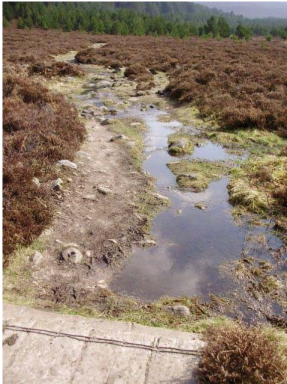
Section 3 – path line gradually migrating down hill.
