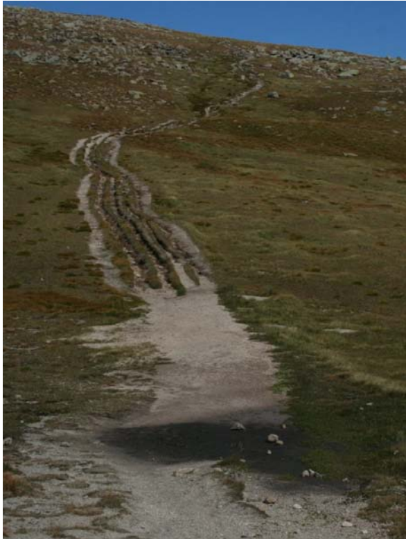
Bad braiding needs contained with water bars to protect path surface.
