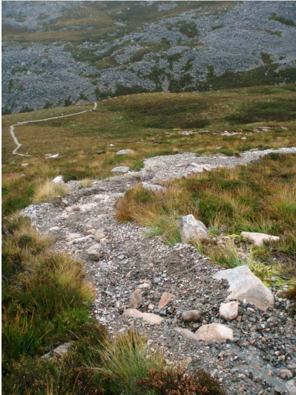
Bad braiding needs contained with water bars to protect path surface.
