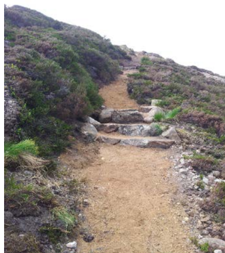
Aggregate surface with anchor bars on Braeriach
