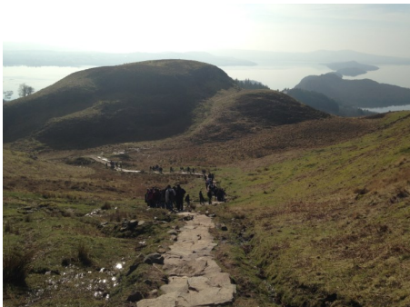
Newly refurbished path at Conic Hill, West Highland Way
