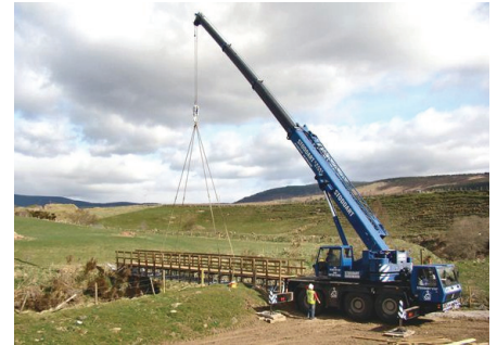
Footbridge being installed at Tarland to Aboyne
